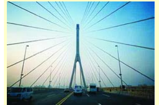
Nanpu and Yangpu Bridges in Shanghai
